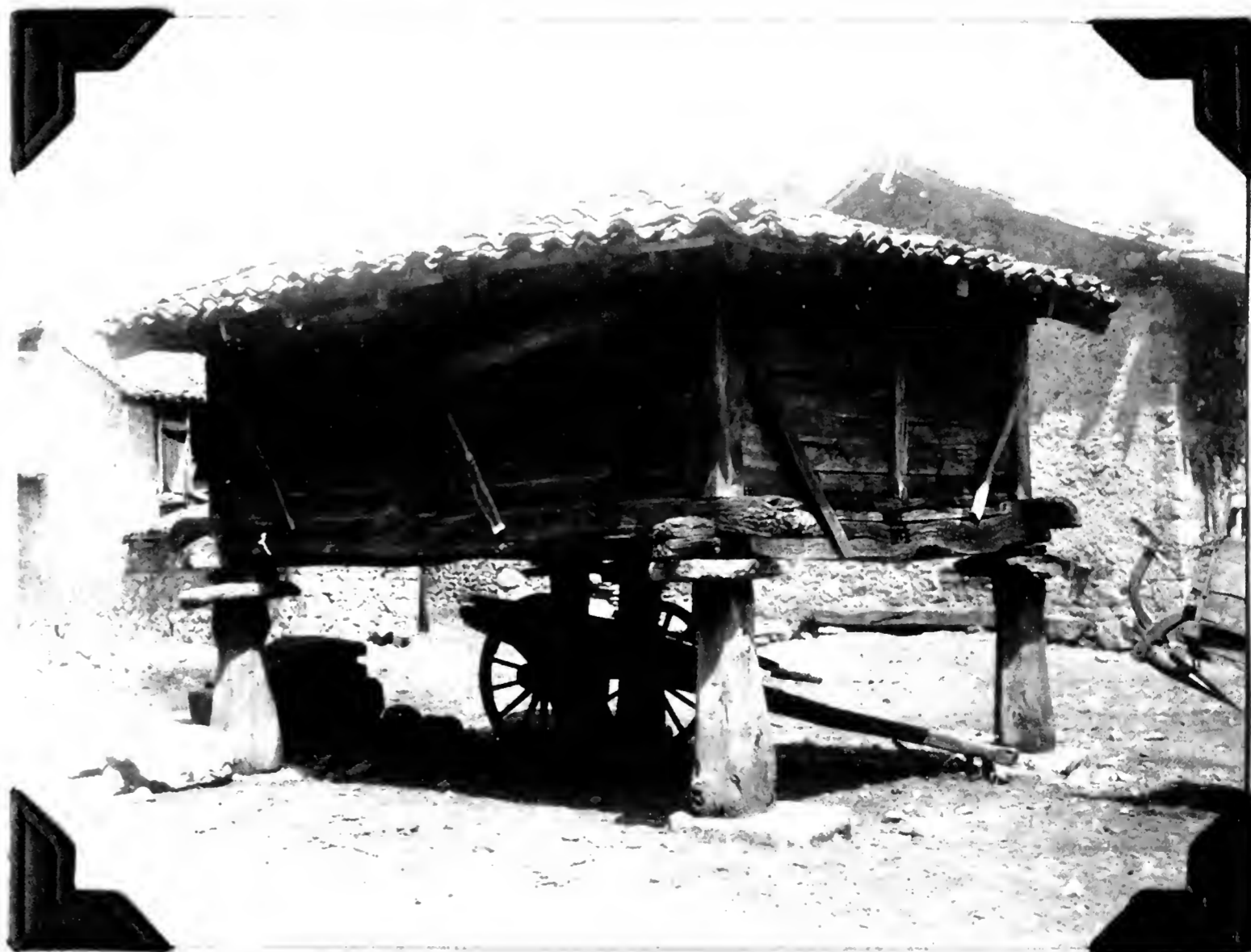
2027. Storehouse for grain in Riaño, León. Note flat stones under corners to prevent climbing rats from entering. May 18, 1930.
